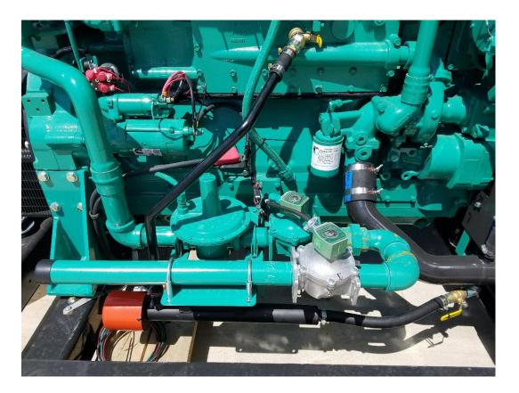
**Spec Note** Check the site fuel pressure and ensure that it meets the generator set fuel supply pressure requirement
