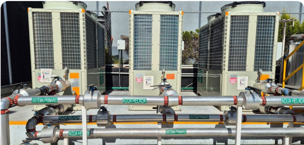
Flexible chiller system at Cummins San Luis Potosí, Mexico, reducing water consumption by over 600,000 gallons annually through advanced cooling efficiency.
