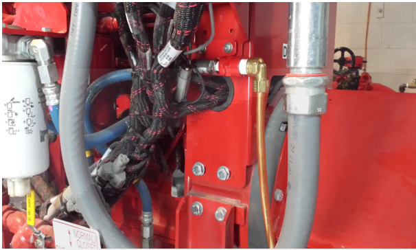
Figure 3-8 VSPLC Pressure Sensing Connection (optional)
